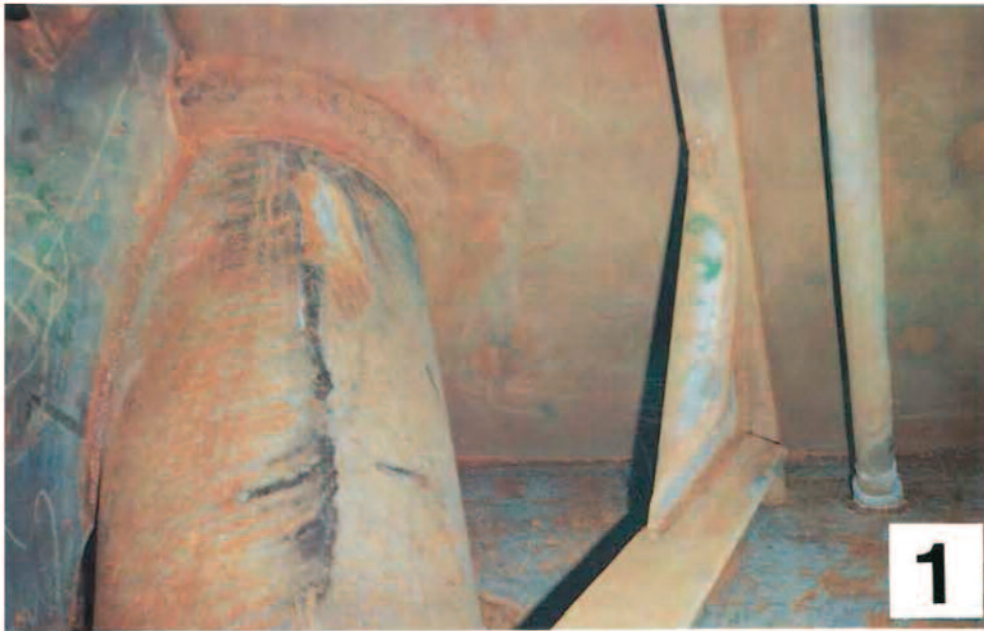
Photo 1. Surfaces prepared for FLUID FILM Gel B (new construction).
