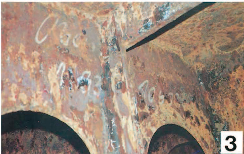
Photo 3. Surfaces prepared for: FLUID FILM Liquid A
