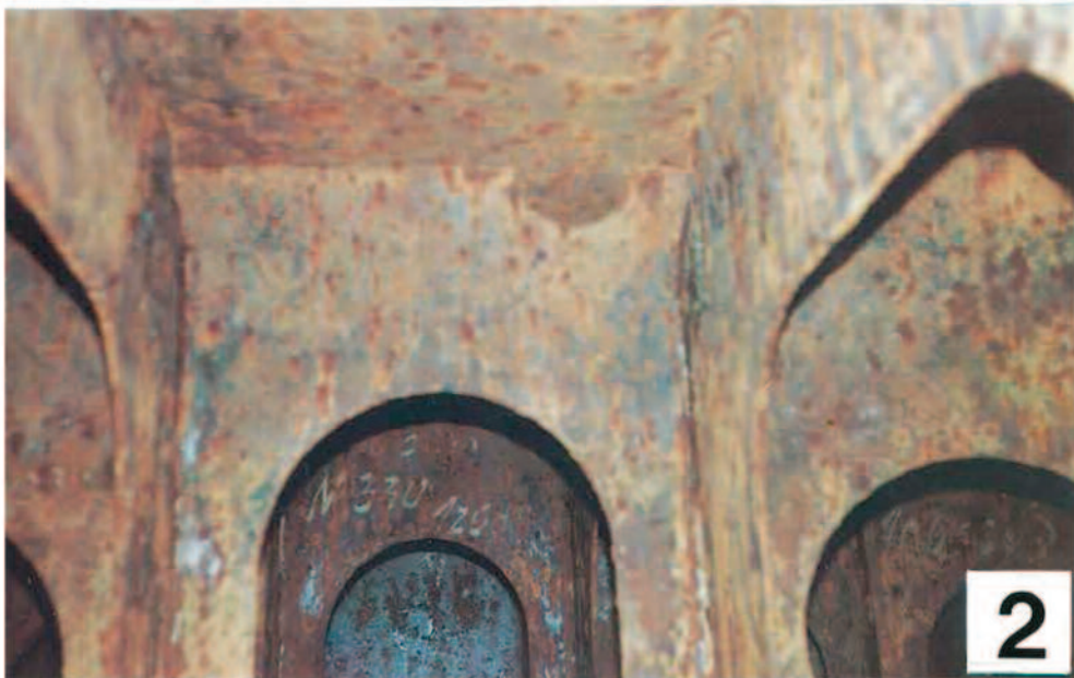
Photo 2. Surfaces prepared for: FLUID FILM Gel B FLUID FILM Liquid AR FLUID FILM Liquid A
